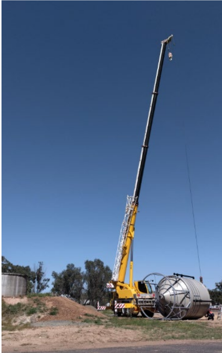
Figure 1: A crane lifted the tank into position
