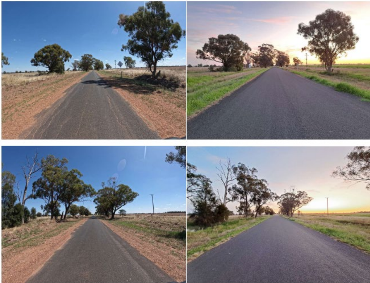
Figure 7: Before (left) and after (right) of Tomingley West Road
