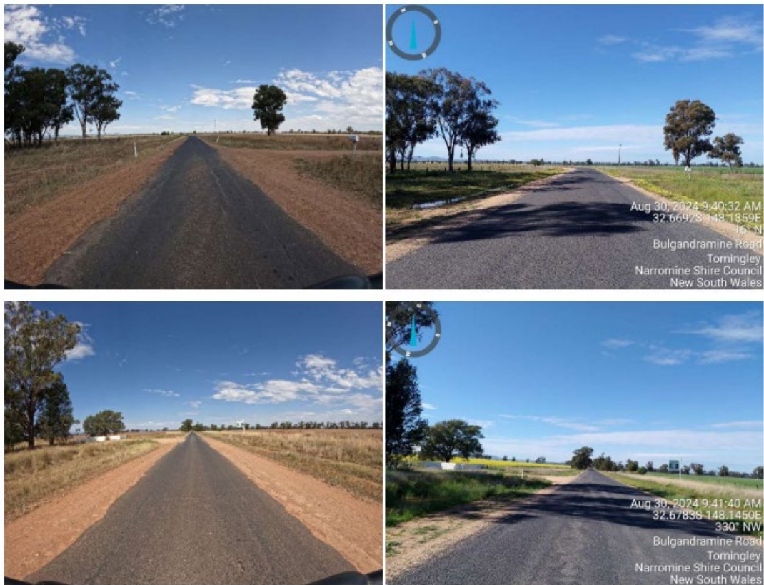
Figure 9: Before (left) and after (right) of Bulgandramine Road
