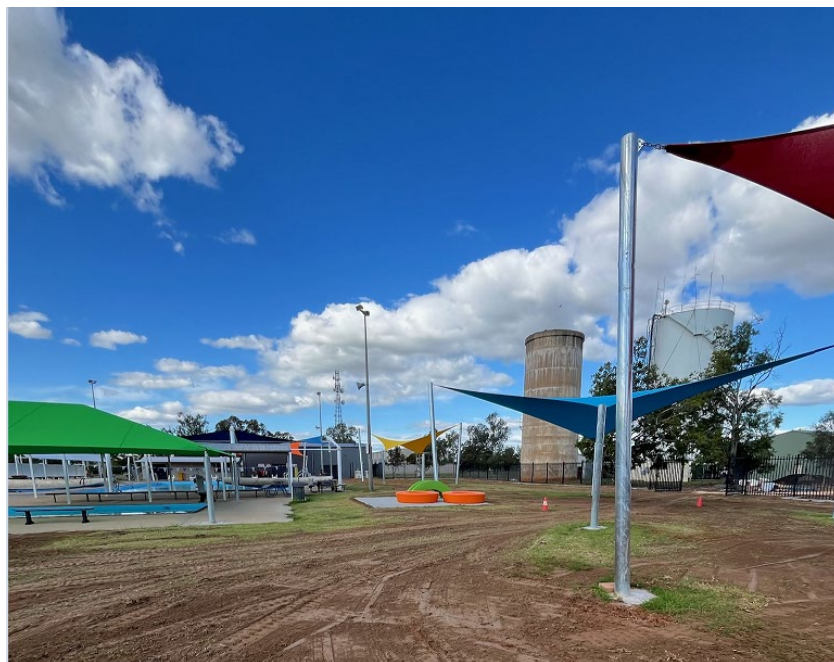
Figure 5: New Shade Sails at the Narromine Pool
