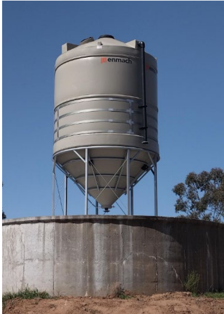
Figure 2: The new reservoir is mounted on top of the existing reservoir
