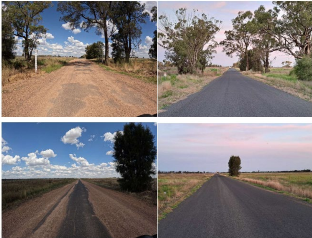
Figure 8: Before (left) and after (right) of Peak Hill Railway Road
